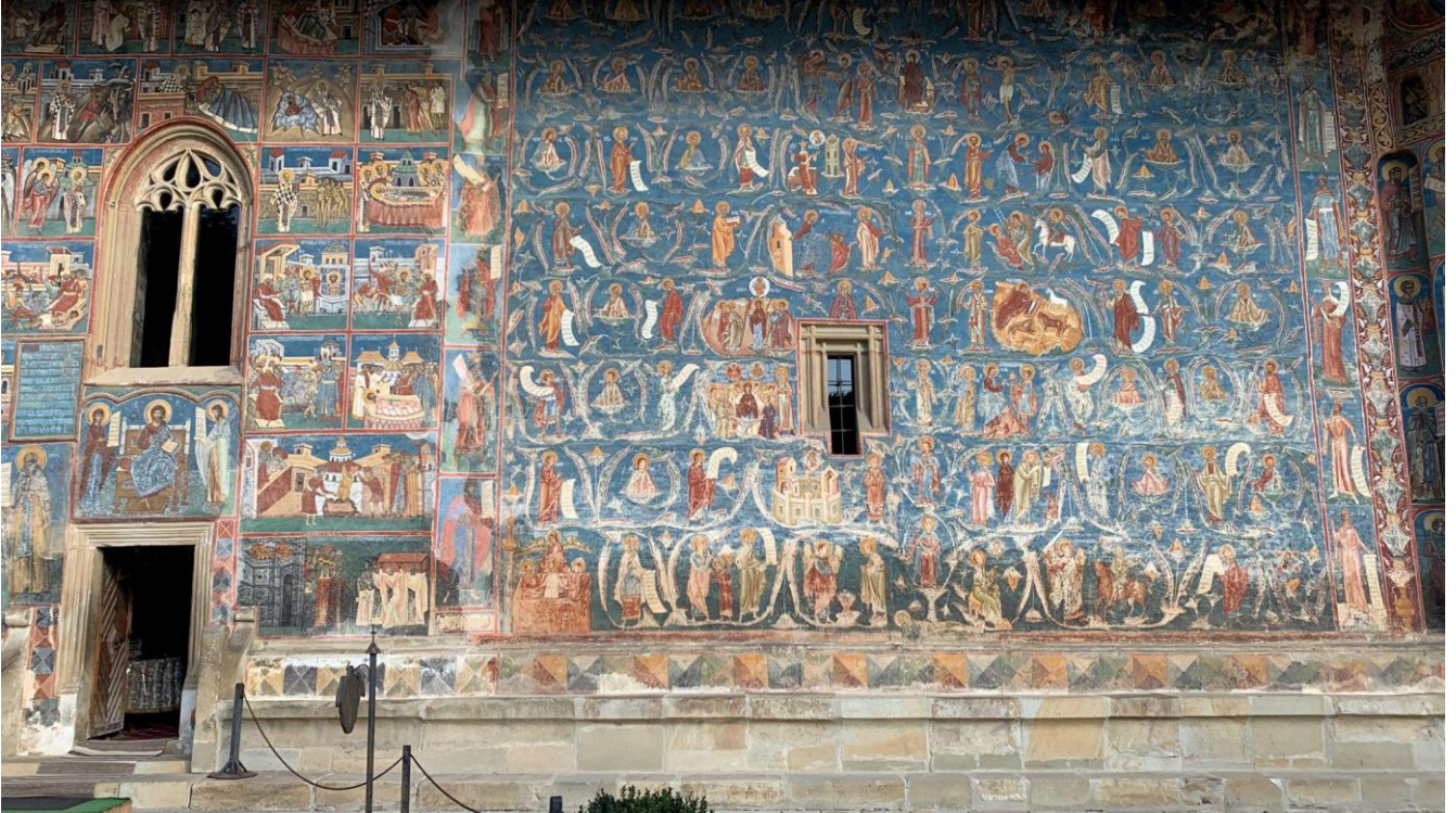
Voronet Monastery Church, South façade, 2022
