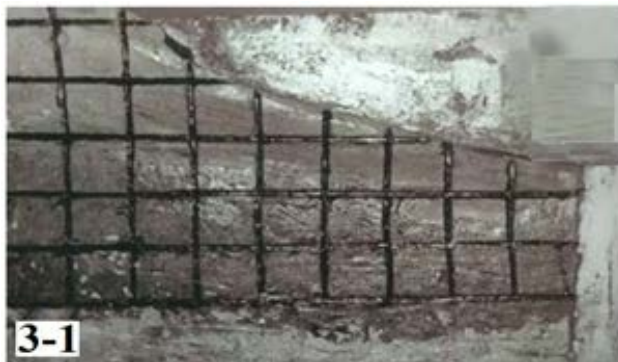
Fig. 15. Model No. 3 before testing. The retaining structure is a solid retaining wall
