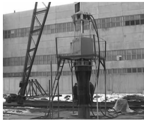
Fig. 1 – Stand for testing a hydraulic hammer (outside view)
