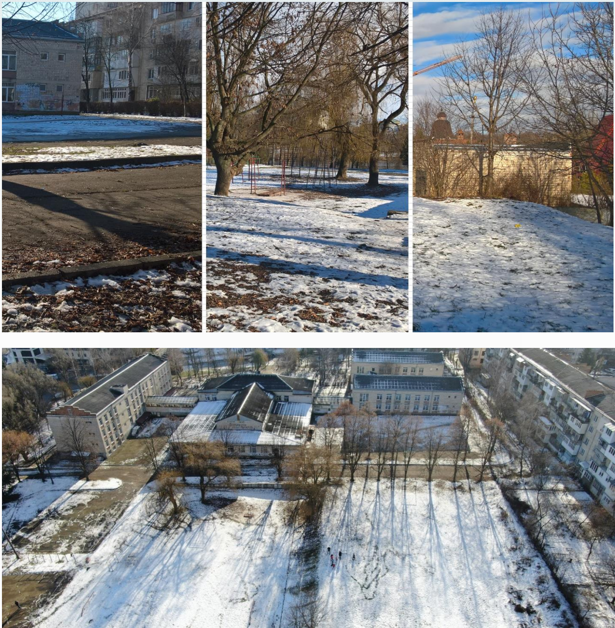
Fig. 2. Situation on the territory of the facility at the time of survey (24.02.2019):
